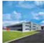
Site Feluy INSULATION
